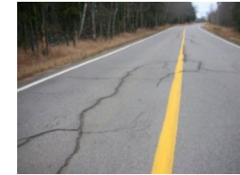
Cracking at low temperature Canada, 2015
