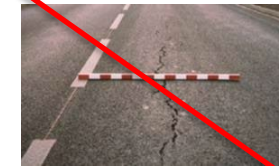
Mechanical fatigue with longitudinal cracks
